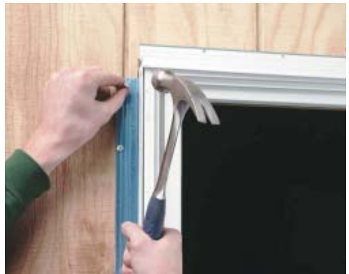
B. Level the window, then fasten the unit in place with roofing nails driven through the nailing flange.
