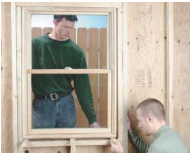
A. Add pairs of tapered shims under the side window jambs and under the center of the sill.
